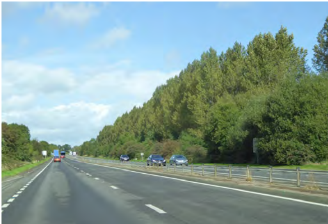
Protihluková bariera v Lancashire (UK)
